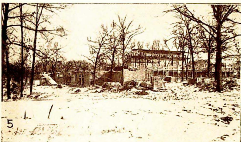
Steel Framework of Assembly Hall Completed, 1924.
